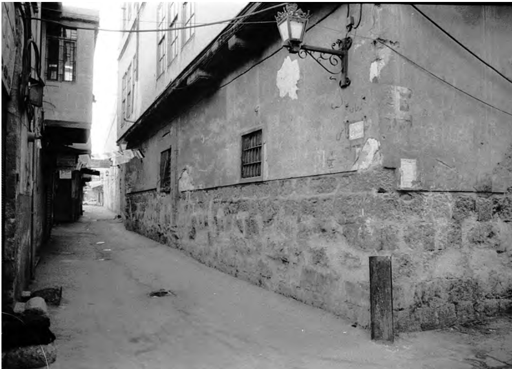
Fig. 7. Damascus, Tankizīyah: east façade
